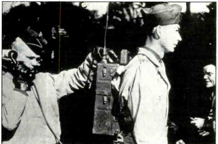
Motorola's SCR-300 'walkie-talkie' was the first two-way FM portable radio. It went into service 50 years ago.
